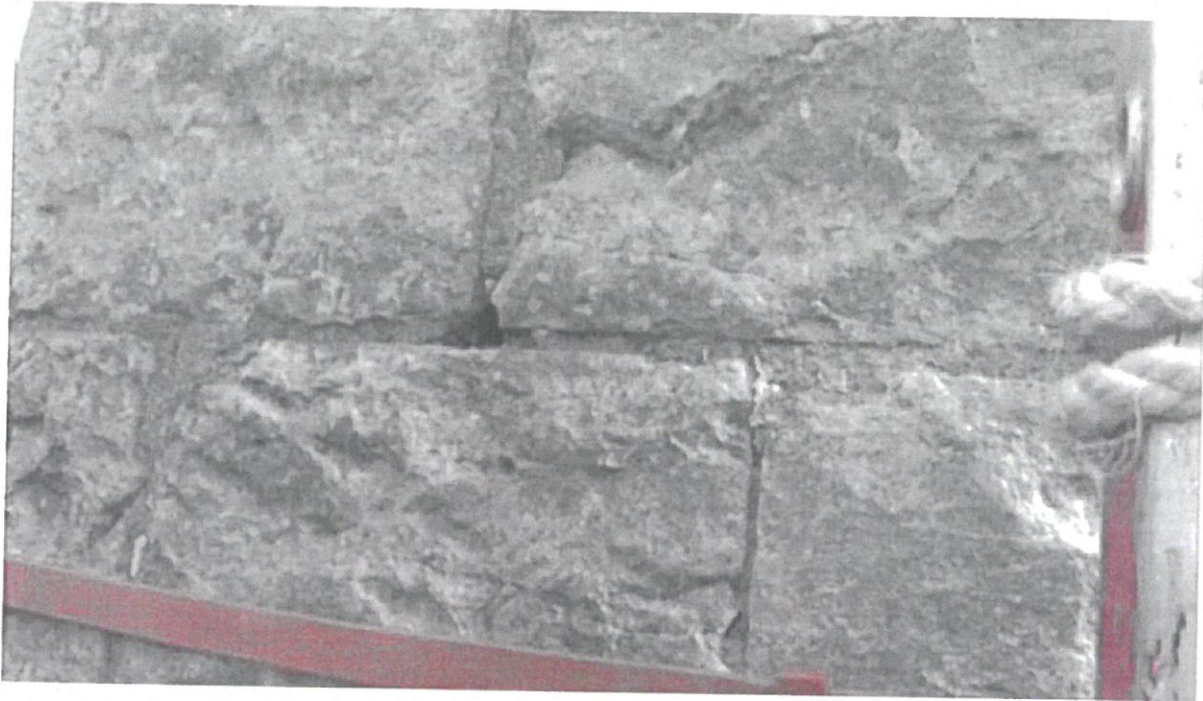
The spire section shows a number of areas where the pointing has failed.
